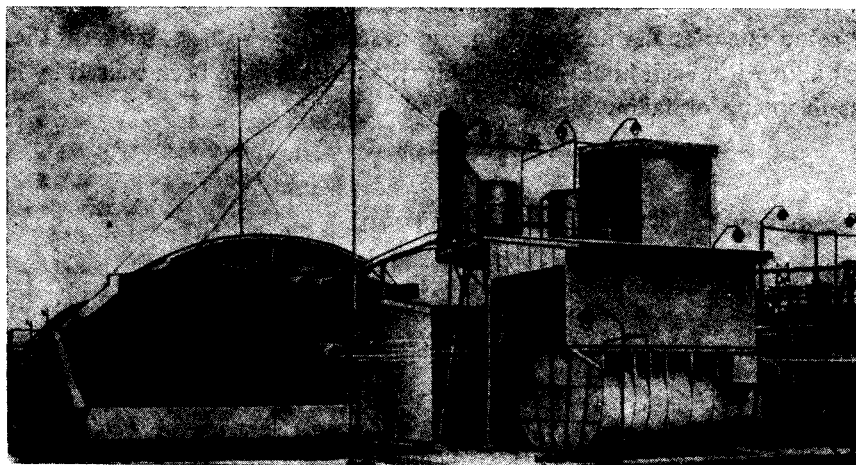
FIG. 64. Nitration Biazzi system building surrounded by earth mound with service tanks in centre and right foreground. The nitration building is protected by lightning arrestors [47]. (I.C.I. of Australia and New Zealand Ltd. at Deer Park, Victoria).
