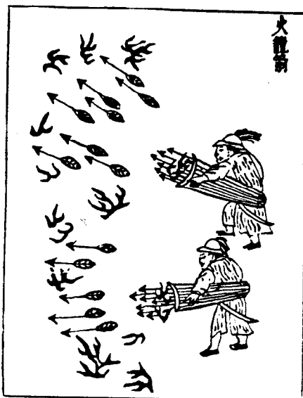
Fig. 1. Incendiary rocket arrows were fired in clusters from round bamboo baskets.
