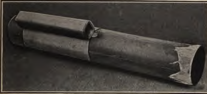
FIG. 30.—Stick-socket binder in place.
