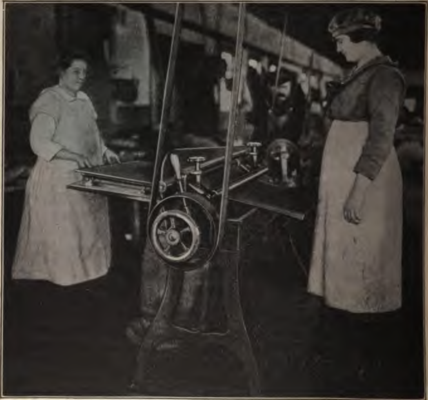
FIG. 87.—Pasting machine.
