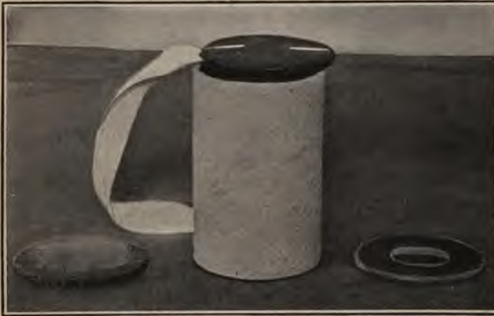
FIG. 185.—Protecting and striker disks.
