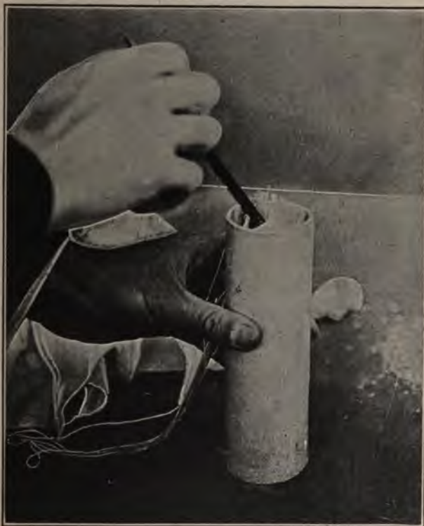
FIG. 61.—Placing cotton batting and sawdust around light in rocket head.
