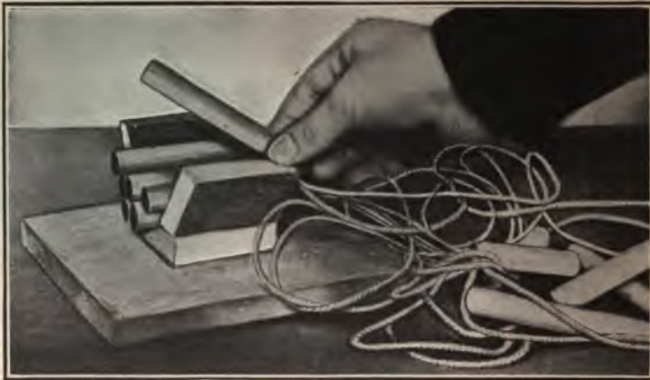
FIG. 58.—Arrangement of caterpillar signals in block.
