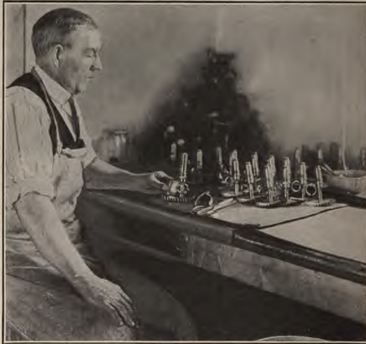
FIG. 127.—Attaching wrapped detonating cap.
