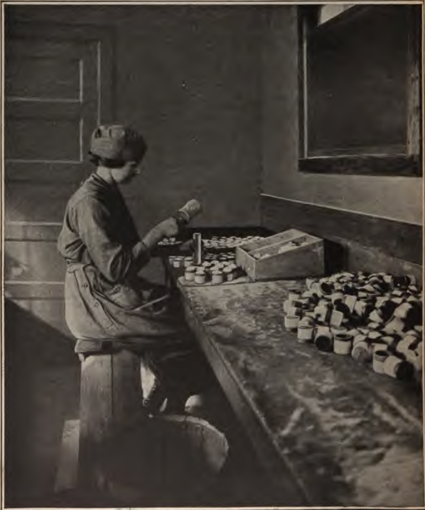
FIG. 144.—Hand loading of light case.
