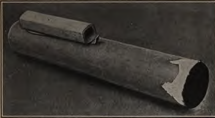
FIG. 29.—Rocket body showing stick socket in place.
