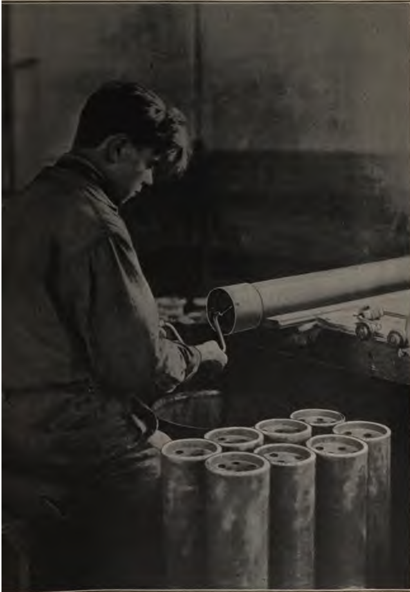
FIG. 99.—Reaming excess composition from loaded case.
