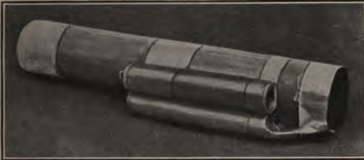
FIG. 38.—Rocket body showing bands and drumhead.
