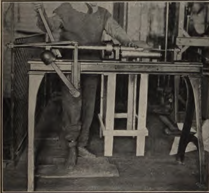
FIG. 6.—Case-rolling machine; feeding paper in slot.
