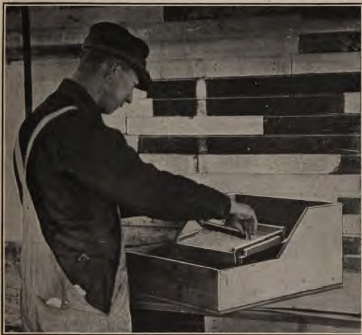
FIG. 179.—Removing excess from measuring frame.
