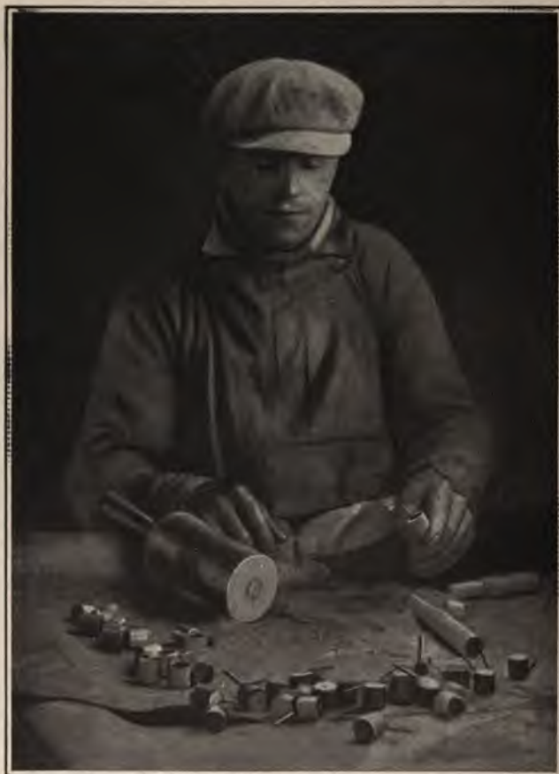
FIG. 159.—Filling light case.
