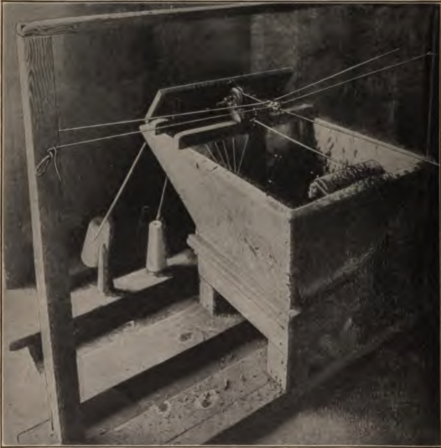
FIG. 103.—Match-making machine.
