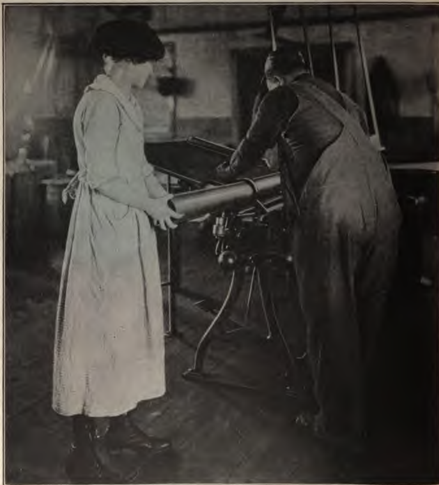
FIG. 89.—Rolling machine; removing case from mandrel.
