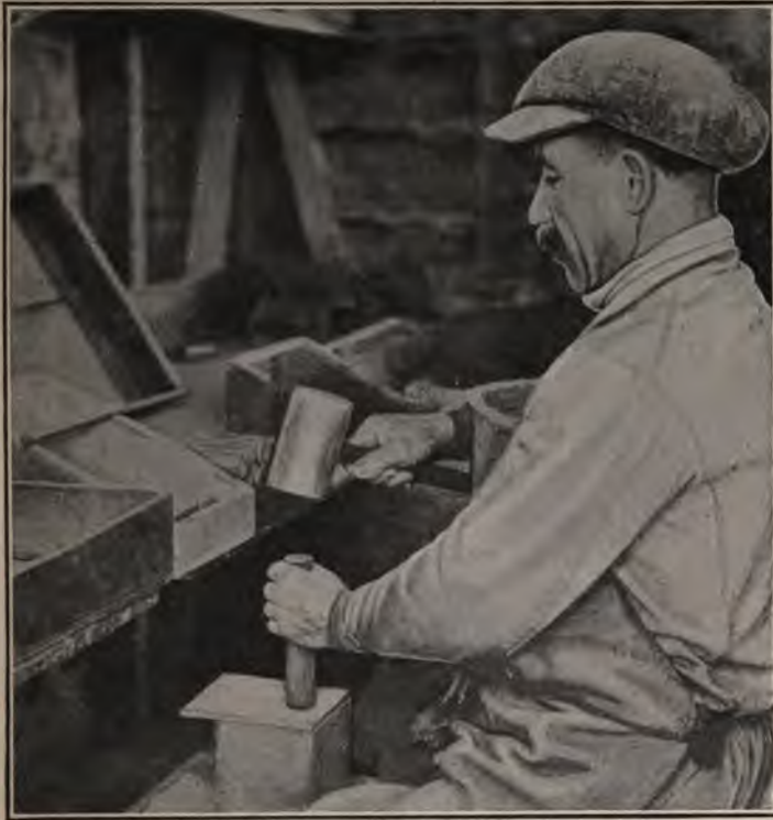
FIG. 51.—Ramming charge into light case.
