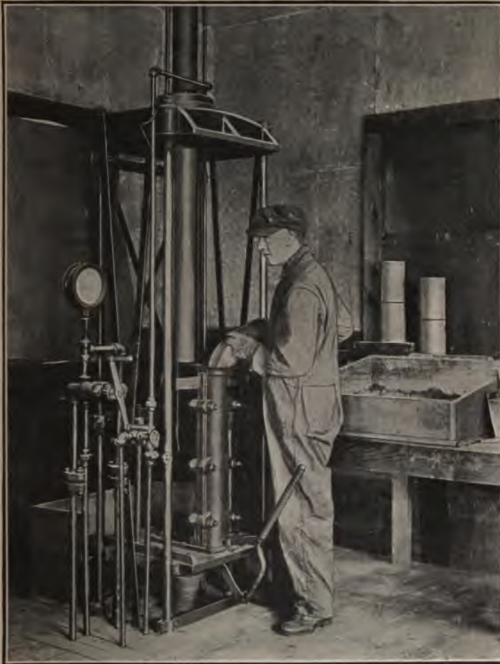
FIG. 96.—Hydraulic press; filling case.
