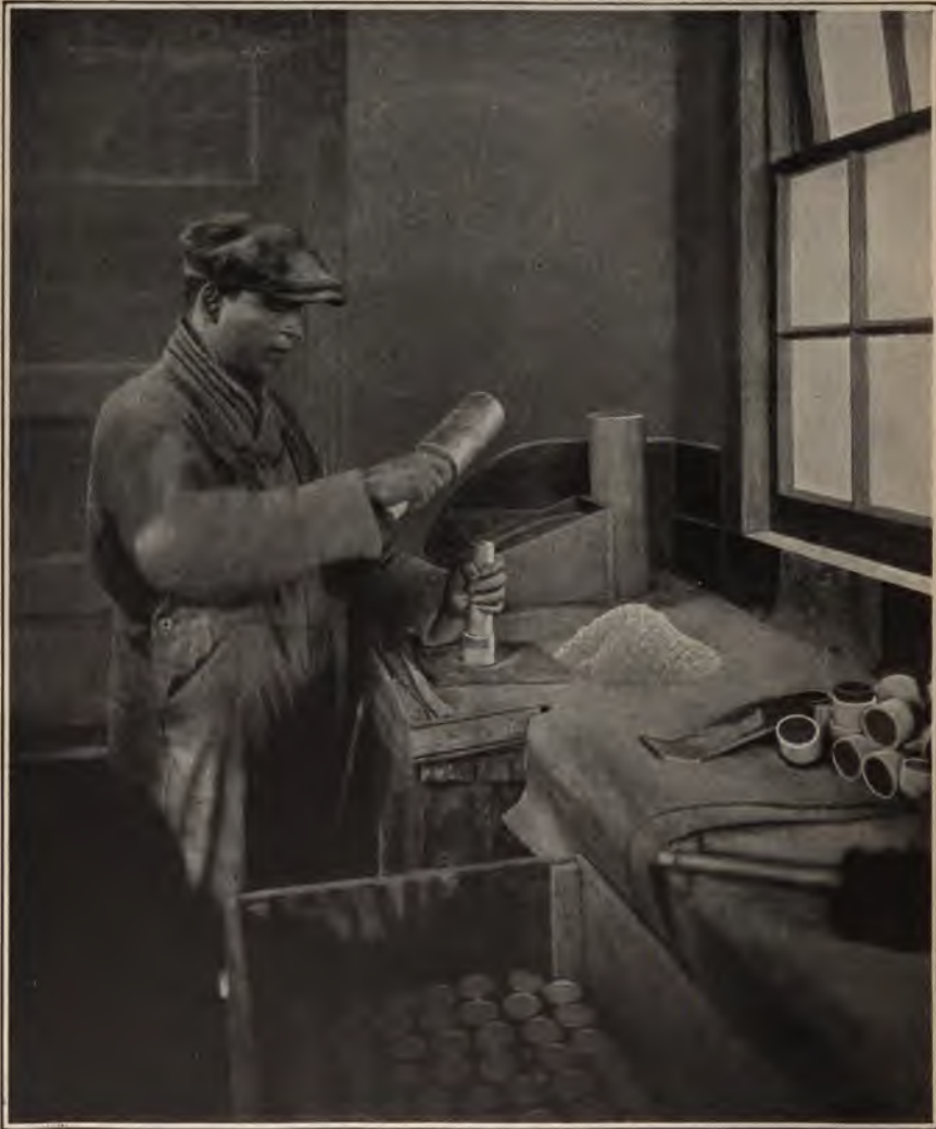
FIG. 163.—Charging red-star light case.
