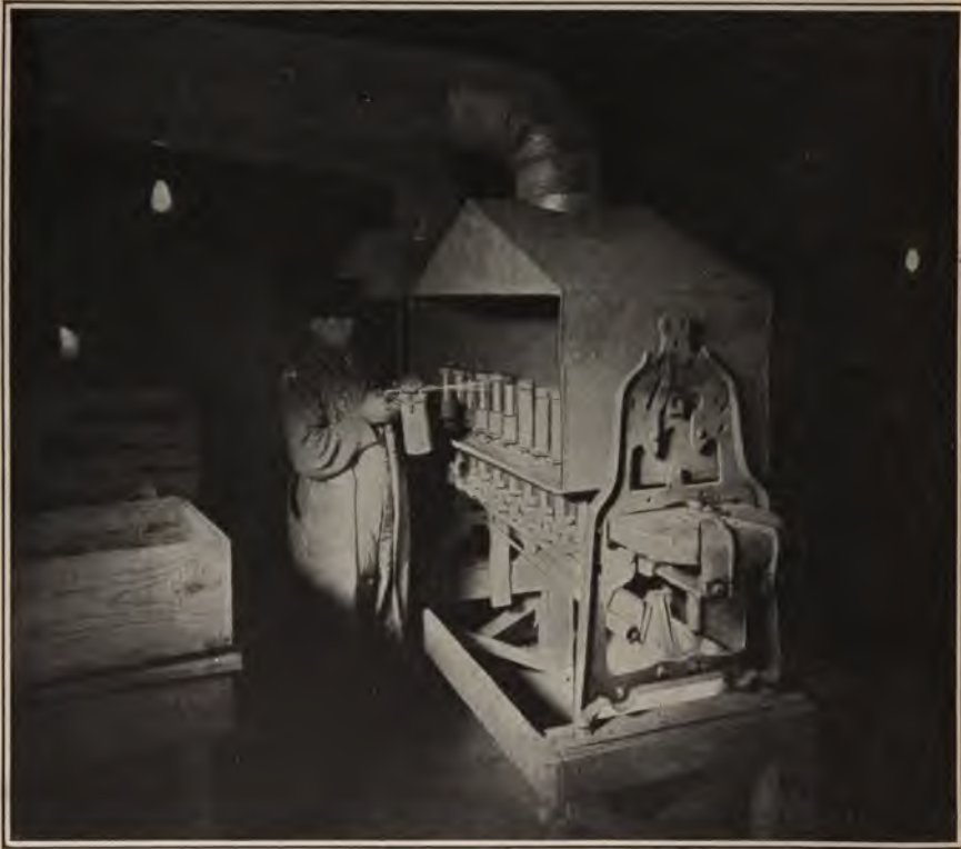
FIG. 138.—Shell-painting machine.
