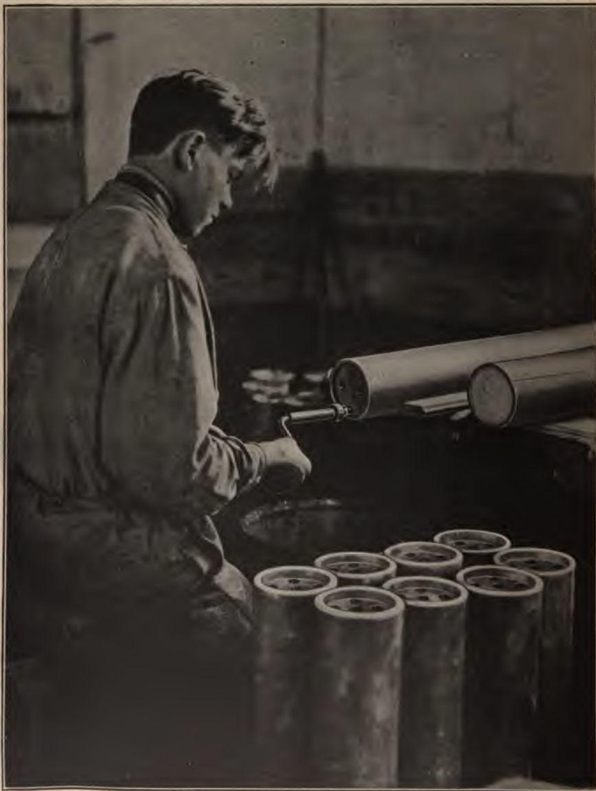
FIG. 100.—Drilling holes in composition.
