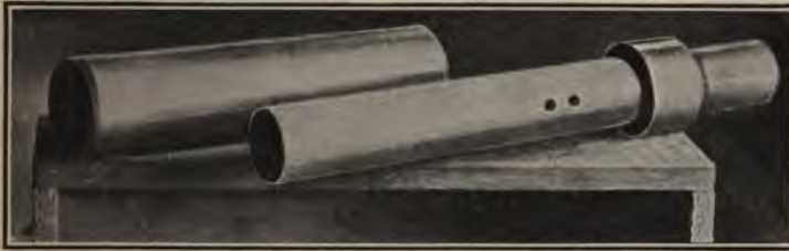
FIG. 42.—Briquette plunger and mold.
