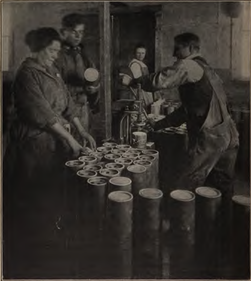
FIG. 101.—Loading first fire in case.
