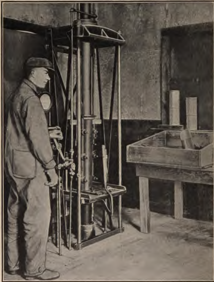
FIG. 97.—Hydraulic press; ramming composition.
