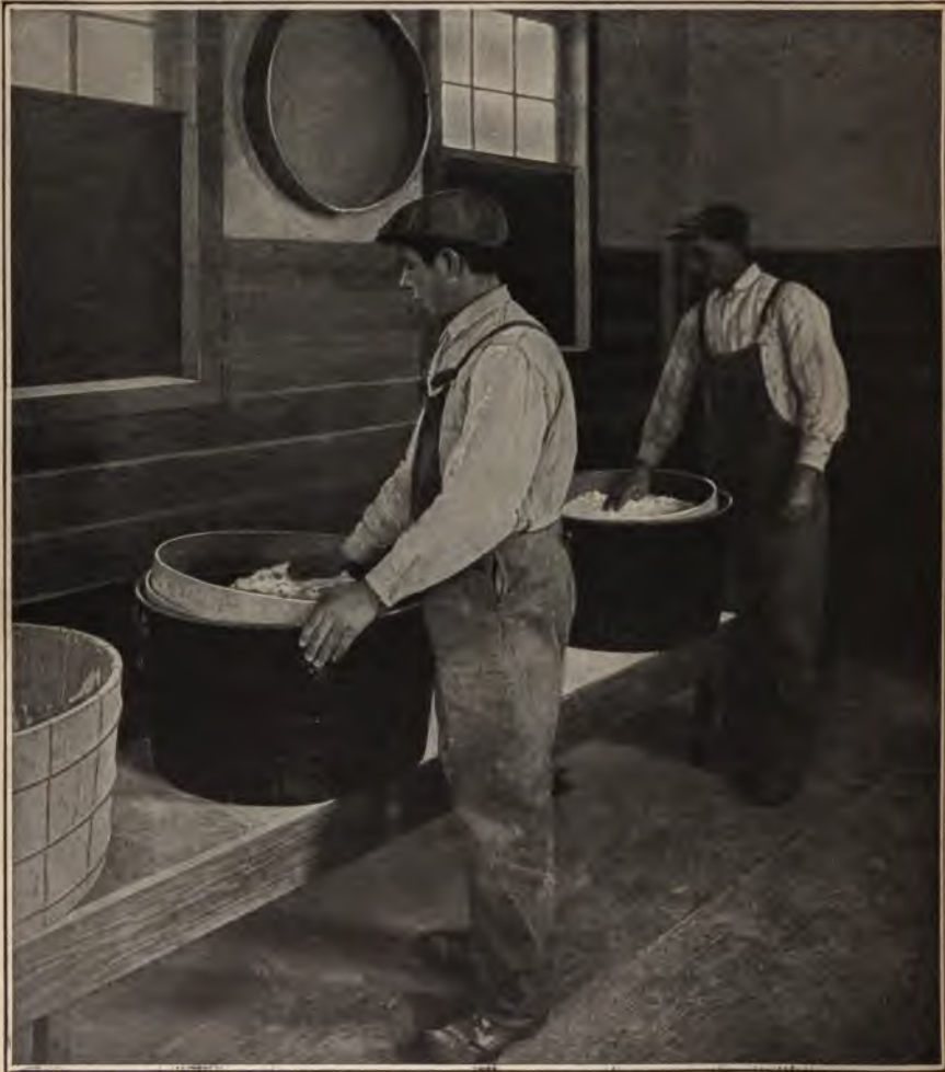
FIG. 143.—Method of mixing composition by hand.
