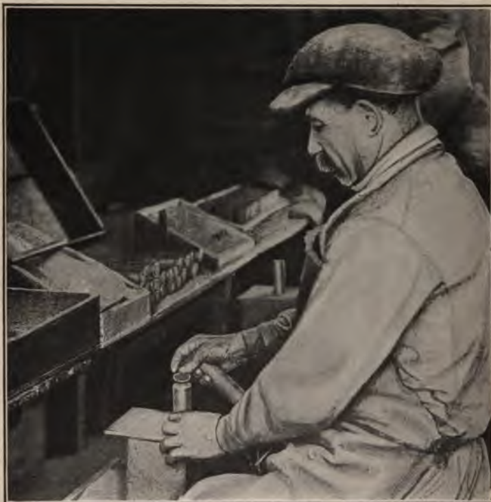
FIG. 52.—Capping light case.
