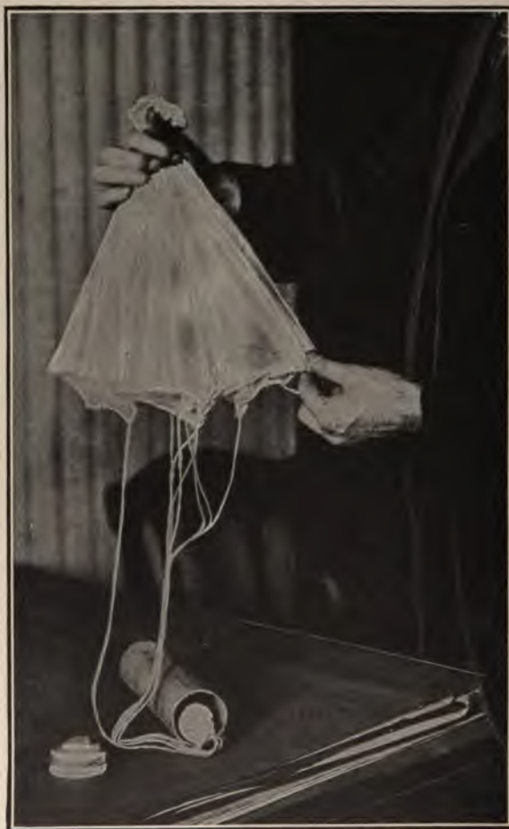
FIG. 149.—Plaiting folds of parachute.
